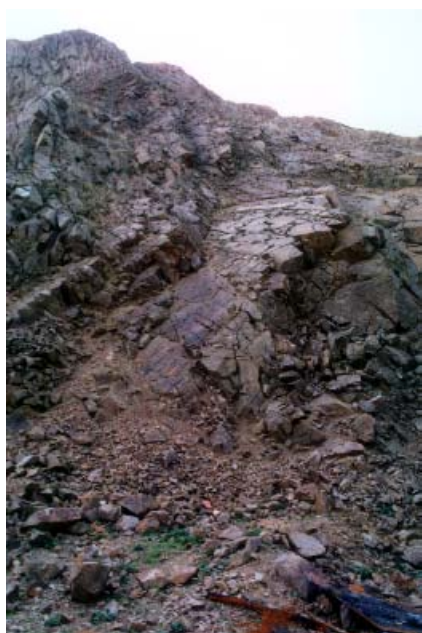
Plate 4 Knock Pike Quarry Structure chutes with debris piles at the foot
