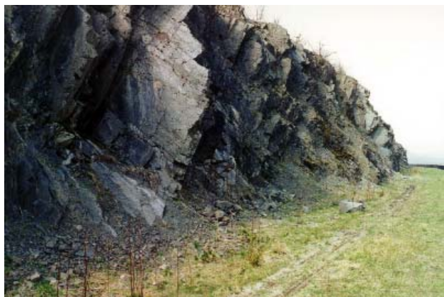
Plate 6 General view of M6 Dillicar showing the range of debris at the slope foot
